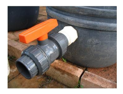
Apply Silicone sealant around the joint inside the tank.
