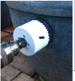
For the bottom outlet, make a hole in the wall of tank approx 20 cm from bottom of the tank. The hole should be a tight fit for the PVC fitting and can be made either by heating a 3"steel pipe and pushing this through the wall or by drilling as shown in the photos.
