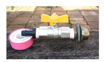
For the top valve fit the threaded fittings together with Teflon plumbers tape. Cut 2 rubber rings the size of the 2 metal washers. Then assemble as mentioned for bottom valve.
