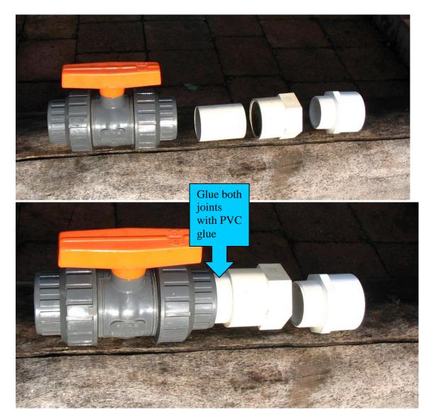
Glue the non threaded PVC fittings together with PVC plumbing glue. Better not to use silicone or Araldite or similar 2 component glues.
